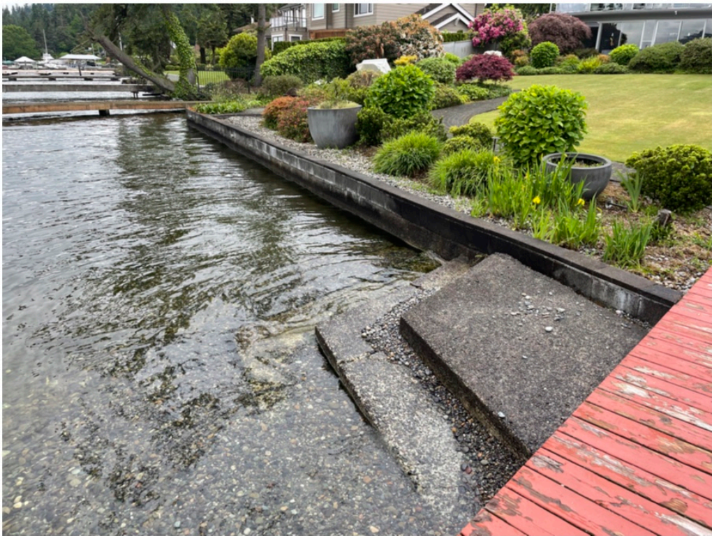
Photo 4 - Shoreline conditions south of dock. Note concrete stairs to be removed.
