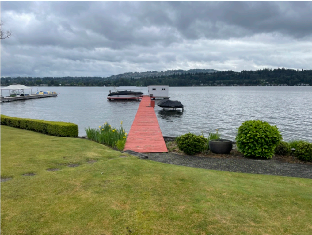
Photo 1 - Existing dock looking waterward.
