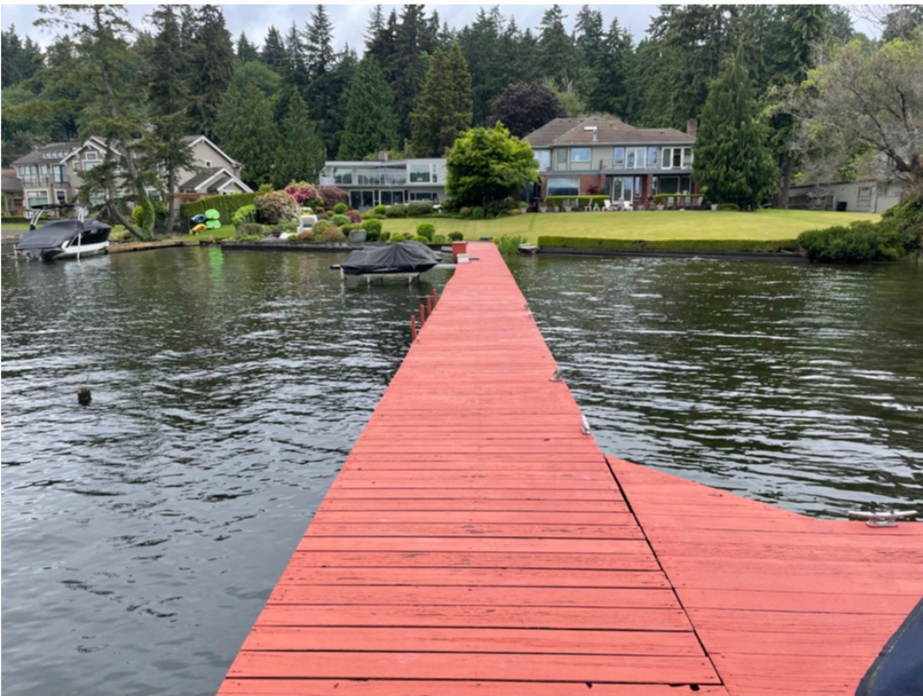
Photo 2 - Existing dock looking landward.
